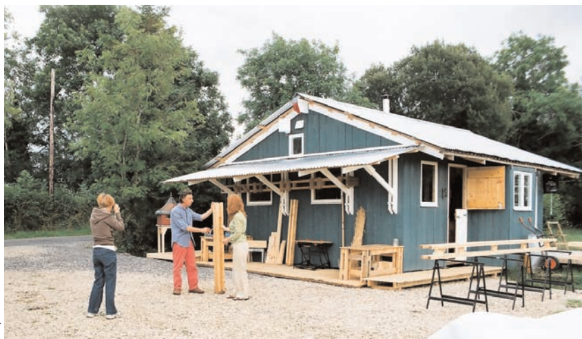
EconoSpace as Site Office & Workshop
