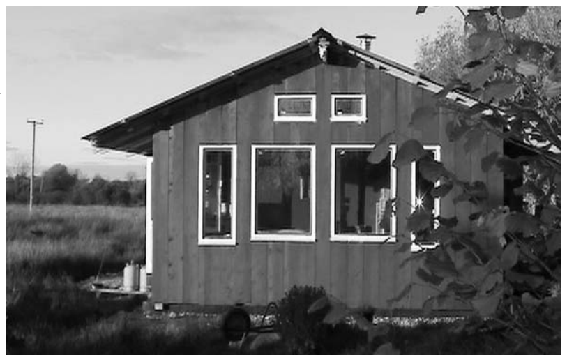
Living Architecture Centre EconoSpace/Site Office
